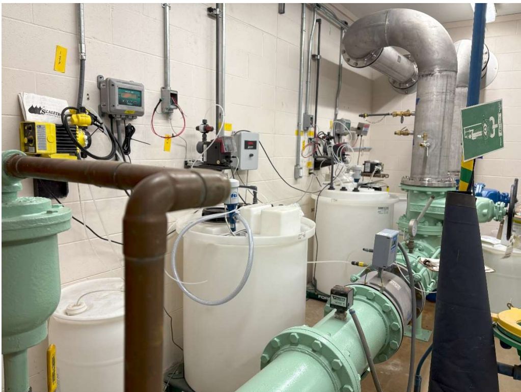
Chemical Feed Equipment Installed
