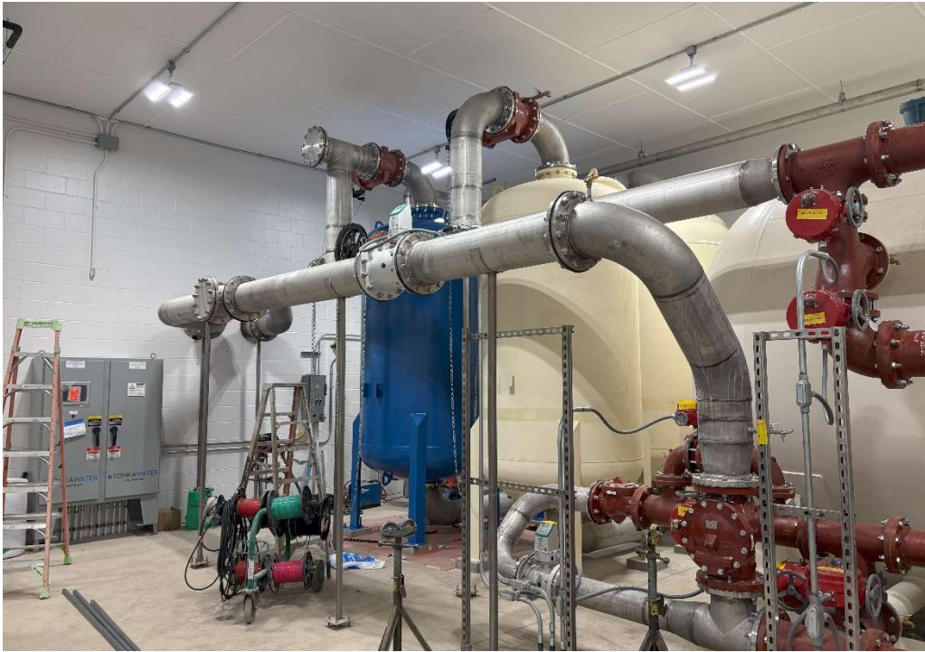
Process Piping Installed
