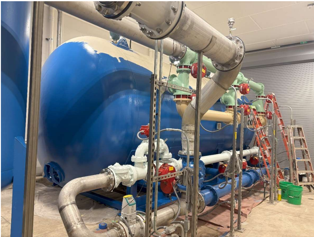
Final Coat of Paint on Horizontal Vessel
