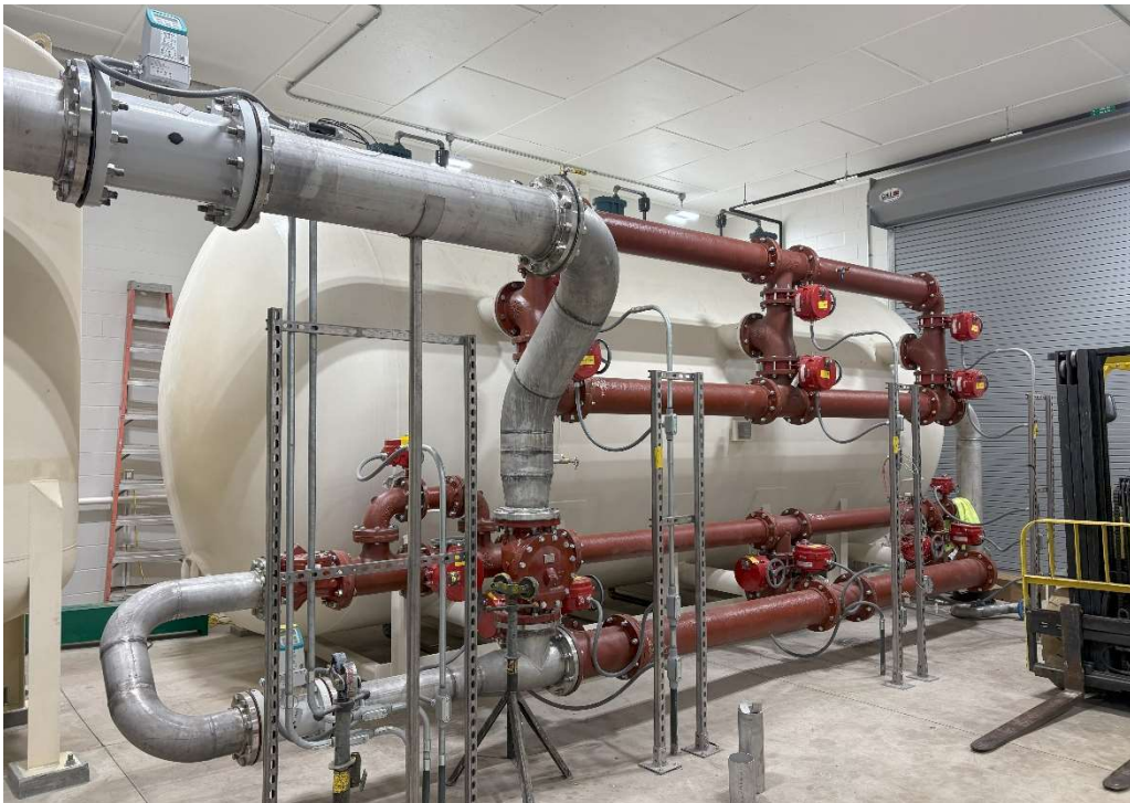
Process Piping Installed
