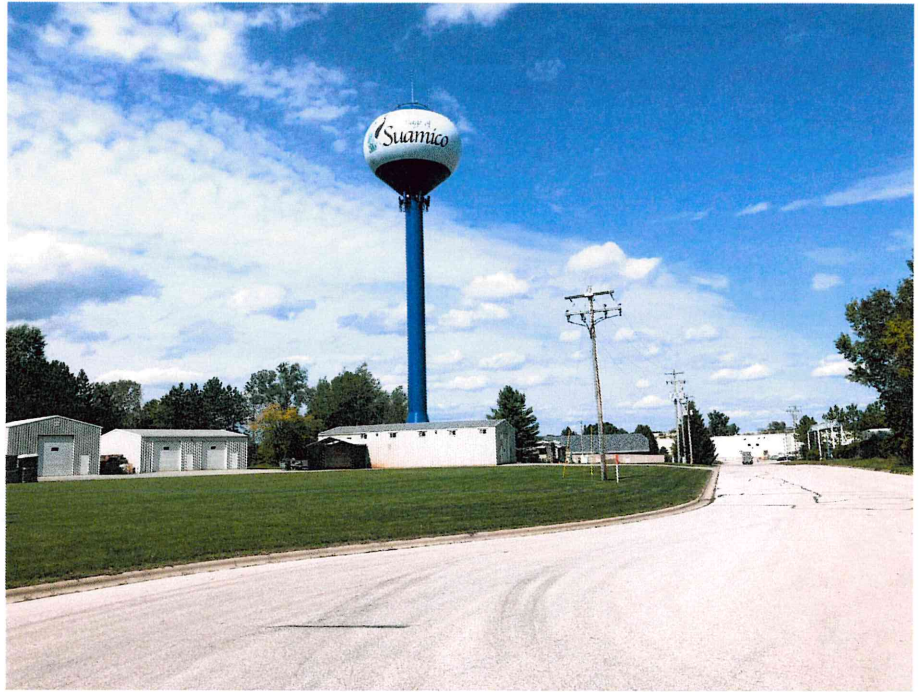
Current Village Water Tower at 1877 Pride Terrace
