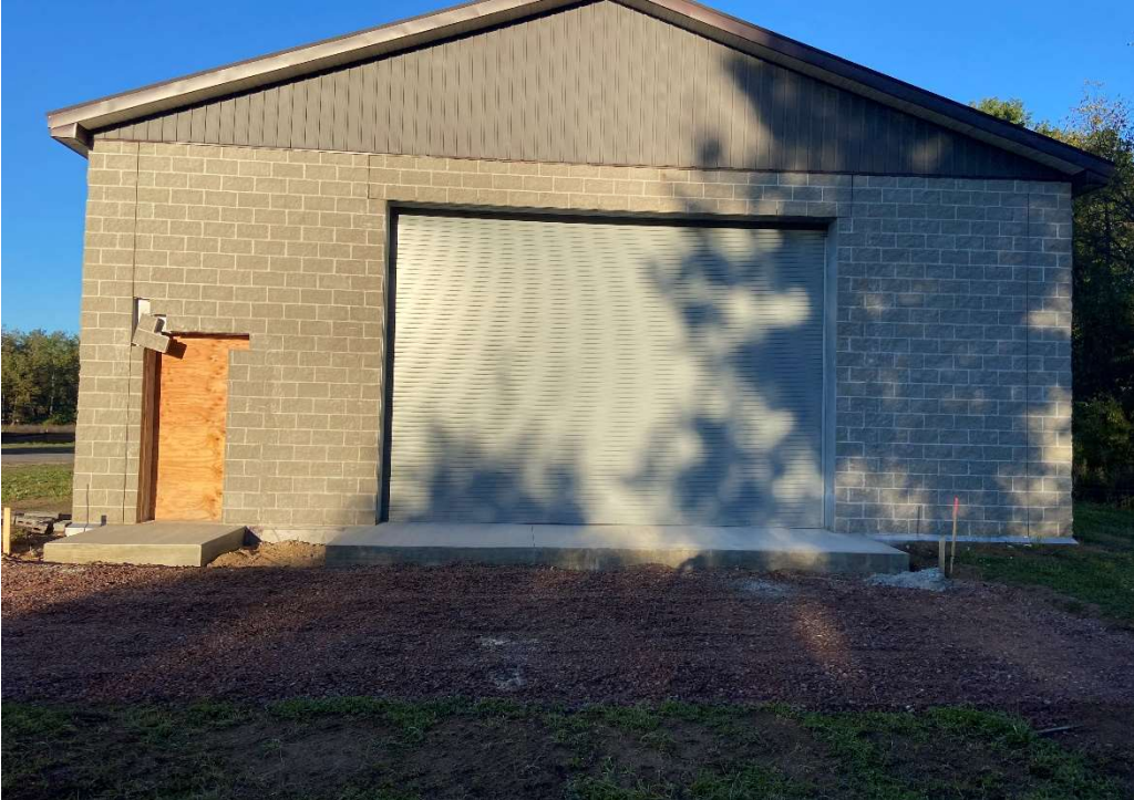
Overhead Door Installation and Approach Slab Finish
