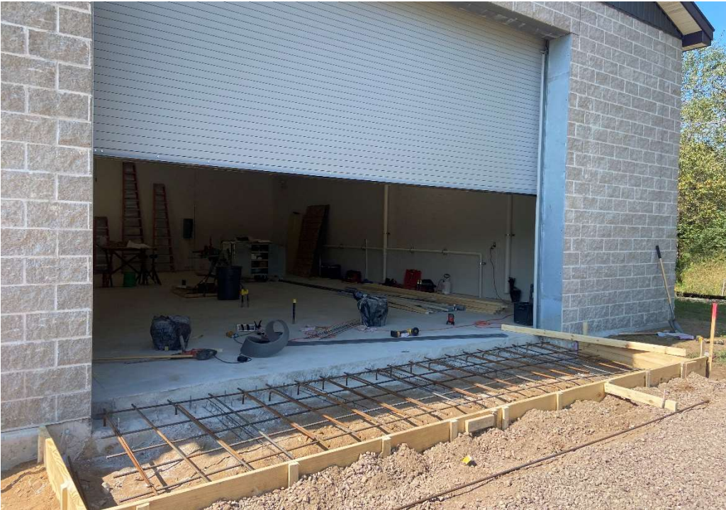
Approach Slab Rebar and Overhead Door Installation
