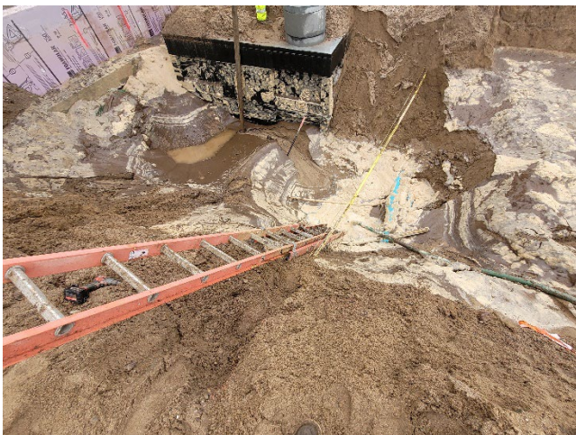
Excavation Hole after Water Pumped Out
