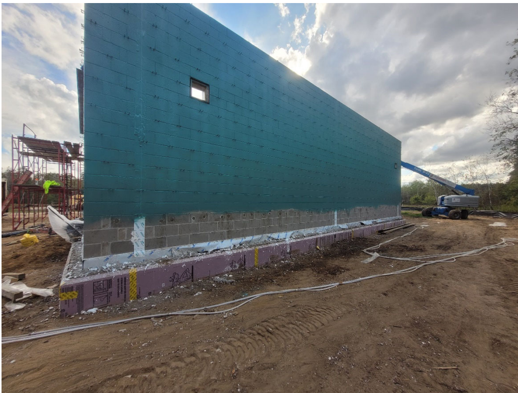
8" concrete masonry unit wall with vapor barrier
