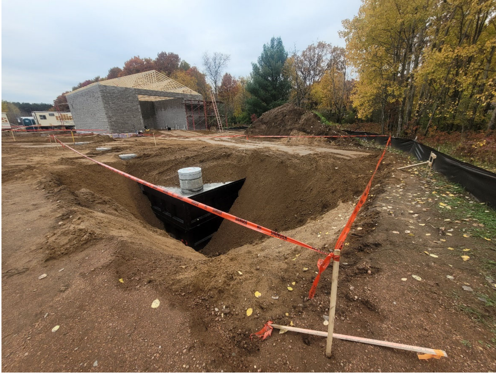
Underground tanks backfilled, trusses installed
