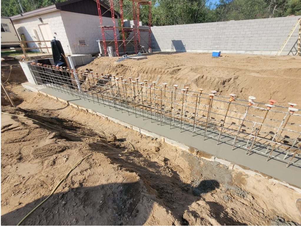
South wall footings, north wall concrete masonry unit walls
