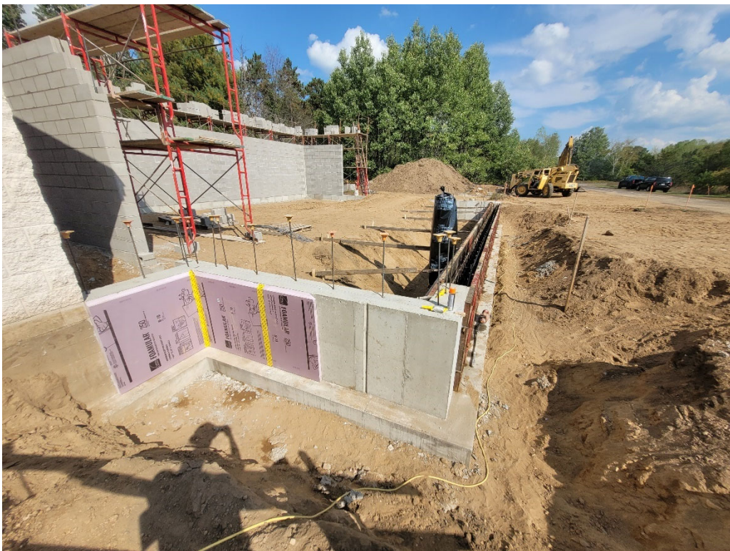
Footings, frost walls, and concrete masonry walls
