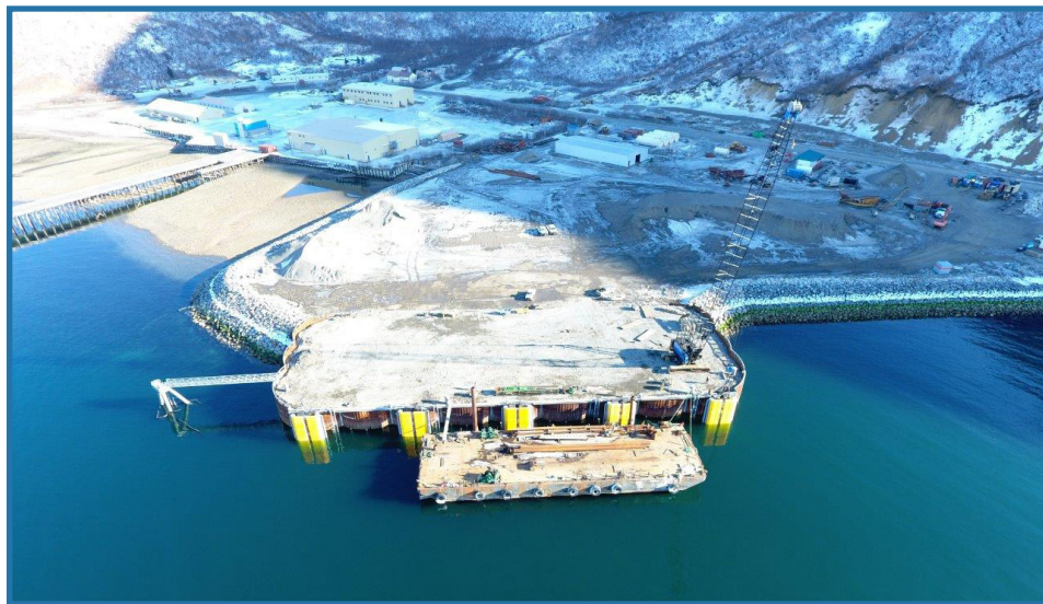
Chignik Dock (under construction)
