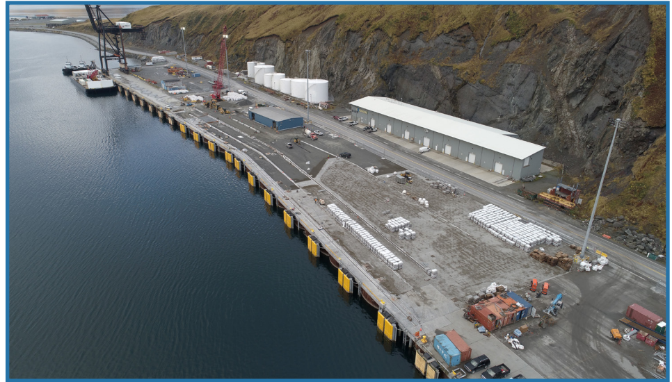
Unalaska Marine Center (during paving)
