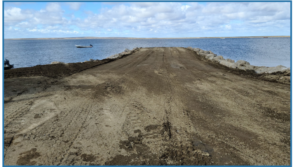
Chefornak Temporary Barge Landing (under construction)
