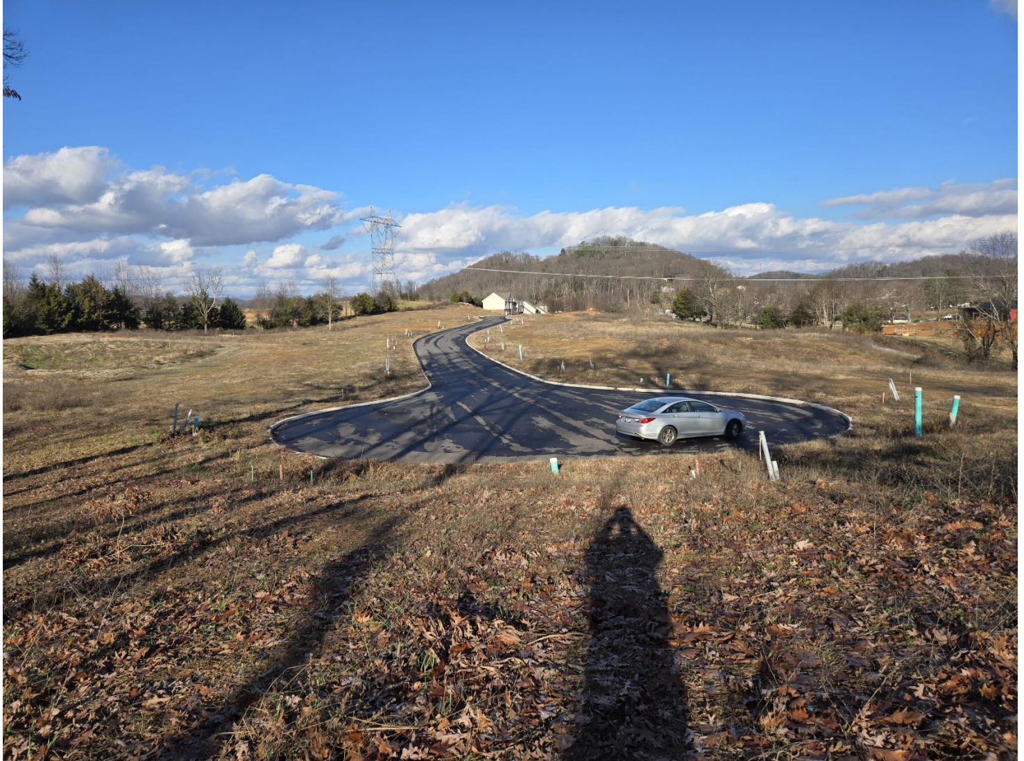
Saint Andrews Garth Phase 3 Eastern View
