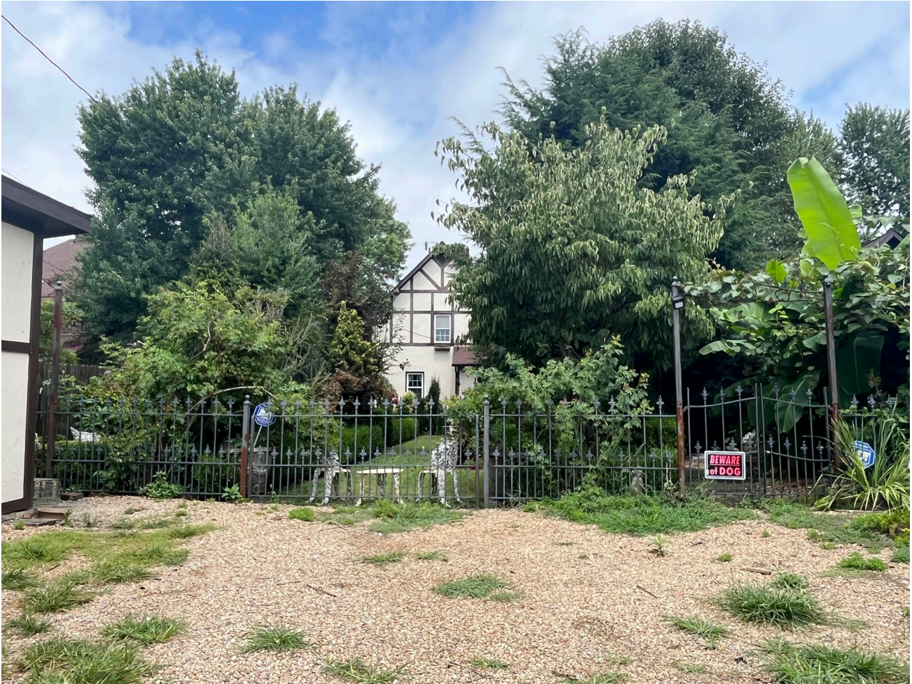
Rear Yard of 209 W Wanola Ave: photo from alleyway
