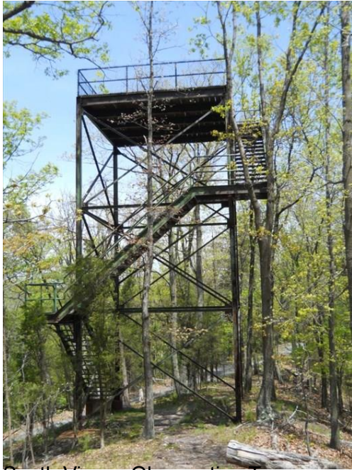
South View – Observation Tower
