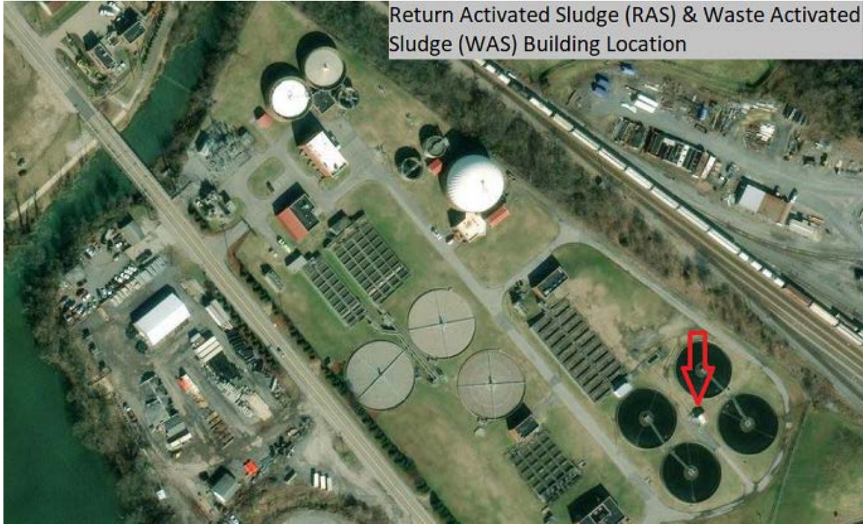
Return Activated Sludge (RAS) and Waste Activated Sludge (WAS) Building
