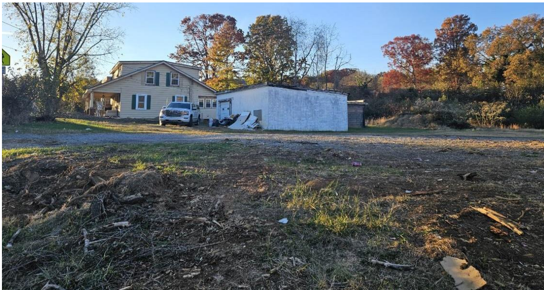
View Toward West
