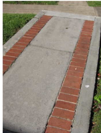
Concrete walk with inlaid brick at 810-812 Yadkin Street.
