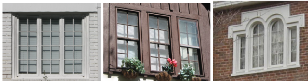
Original casement windows at 809 Yarkin Street.
