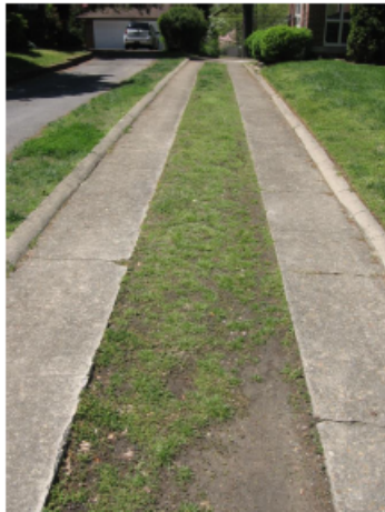
Original concrete ribbon driveway at 1301 Watauga Street.
