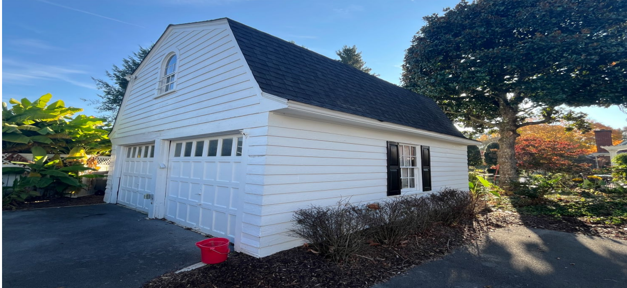
Current Photo of the Garage
