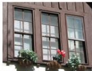
Original four-over-four, wood sash windows at 205 Compton Terrace.
