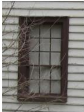
Original nine-over-six wood-sash window at the Netherland Inn.
