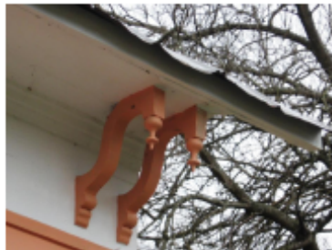
Preserve original wood details such as brackets at 2305 Netherland Inn Road.
