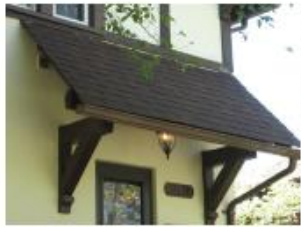
Example of a permanent frame canopy over the entrance at 213 Wanola Avenue.
