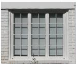
Original casement windows at 509 Tadkin Street.
