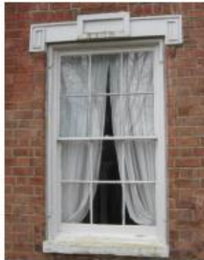
This original six-over-six, wood-sash window with ornamental hood is an important component of Rotherwood.
