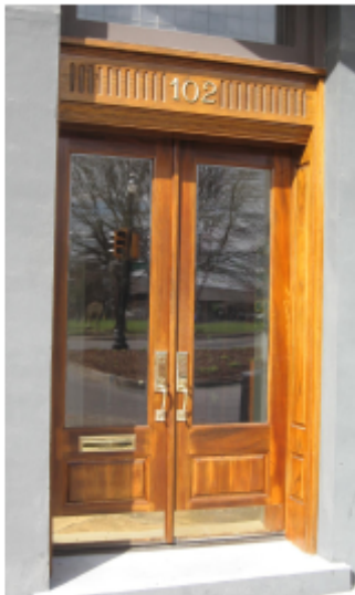
The single-light glass and wood replacement doors at 102 W. Main Street resemble traditional designs and this type of door is appropriate for new doors on Main Street.
