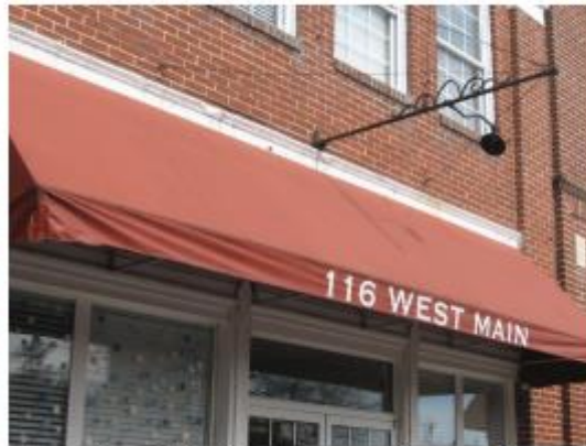
Awning signs with the business name or address are also appropriate on commercial buildings.
