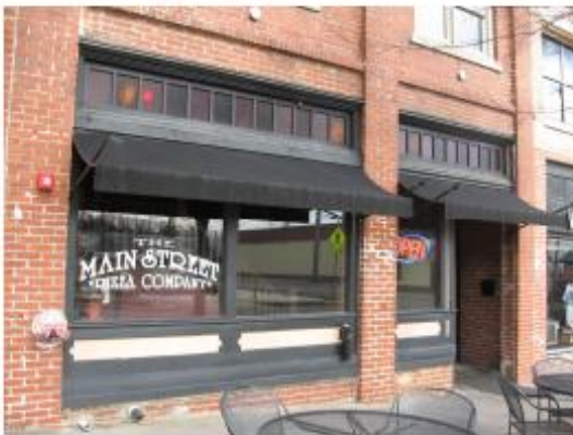
This storefront at 242 E. Main Street retains its original frame bulkheads, display windows and transom.
