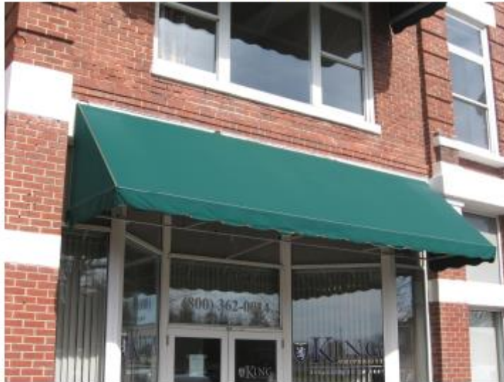
This shed roof canvas awning is an appropriate design at 104 E. Main Street.
