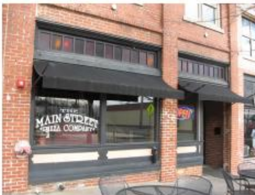
This storefront at 242 E. Main Street retains its original frame bulkheads, display windows and transom.
