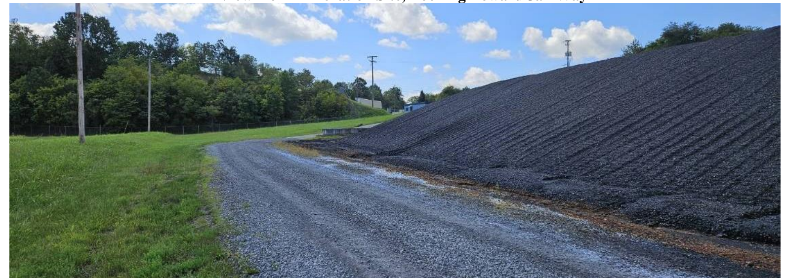
View from Annexation Site, Looking Toward Jan Way
