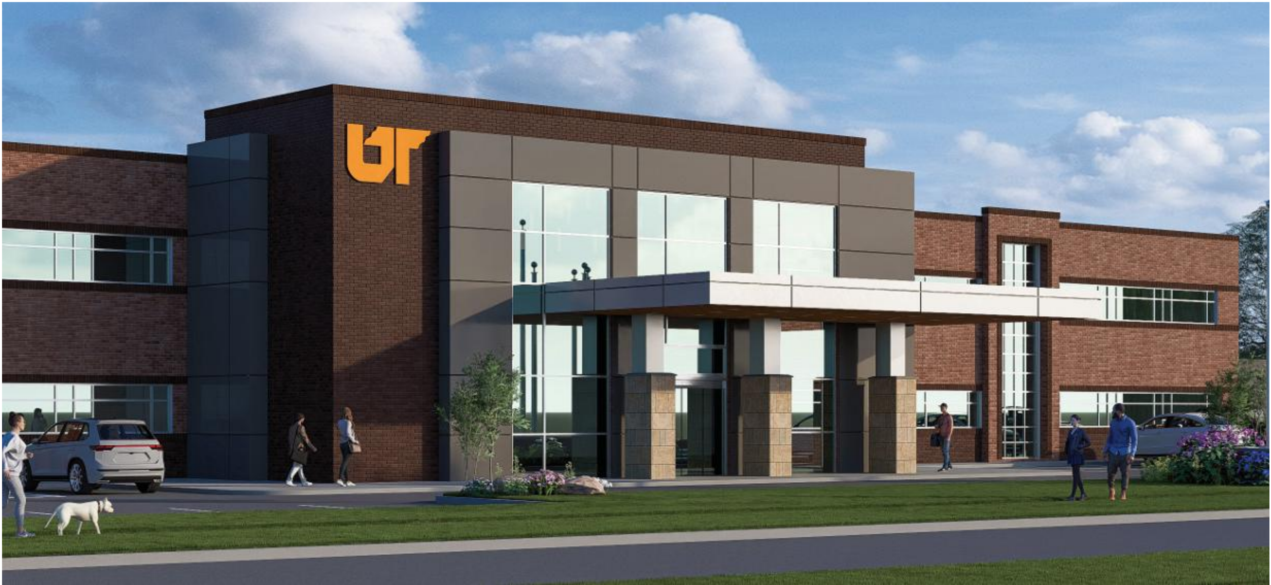
Phase 3 – Exterior renovation provides new entry way, lobby, and second floor student lounge.
