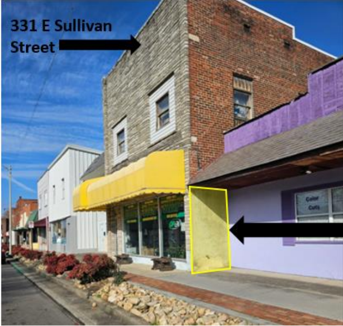
Eastern External Wall Mural Location
