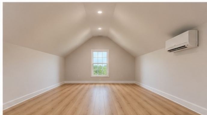
ATTIC – FINISHED WITH SHEETROCK & LVT FLOORING
