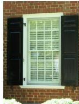
The original twelve-over-twelve, wood sash window at 1261 Watauga Street reflects the dwelling's Colonial Revival style.
