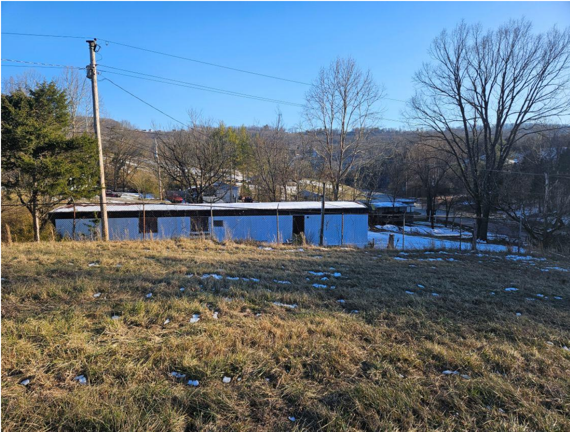
Southern View from Site
