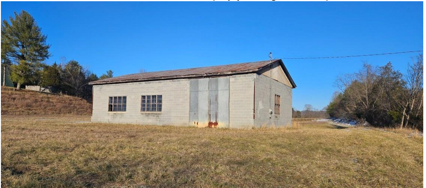
View of Sole Structure on Site (Empty Building to be Razed)
