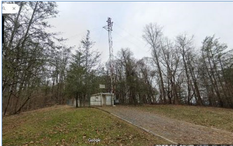
View of Cell Tower from Street
