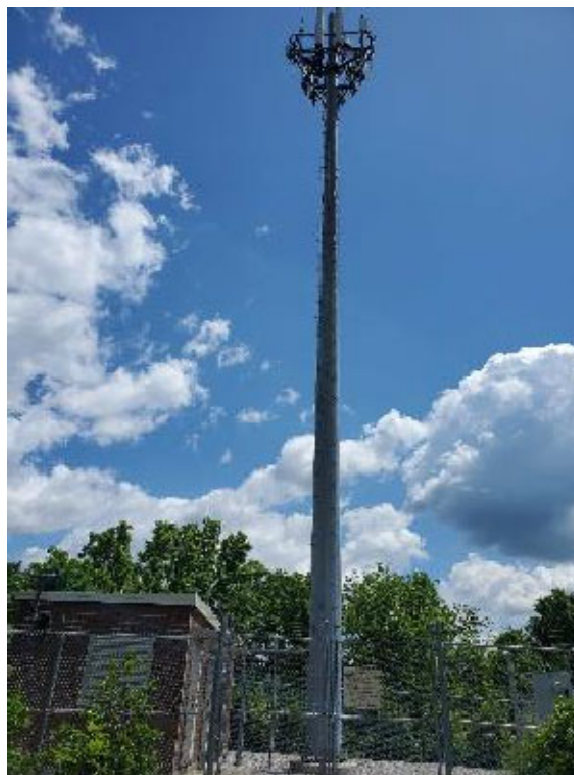
View of Tower
