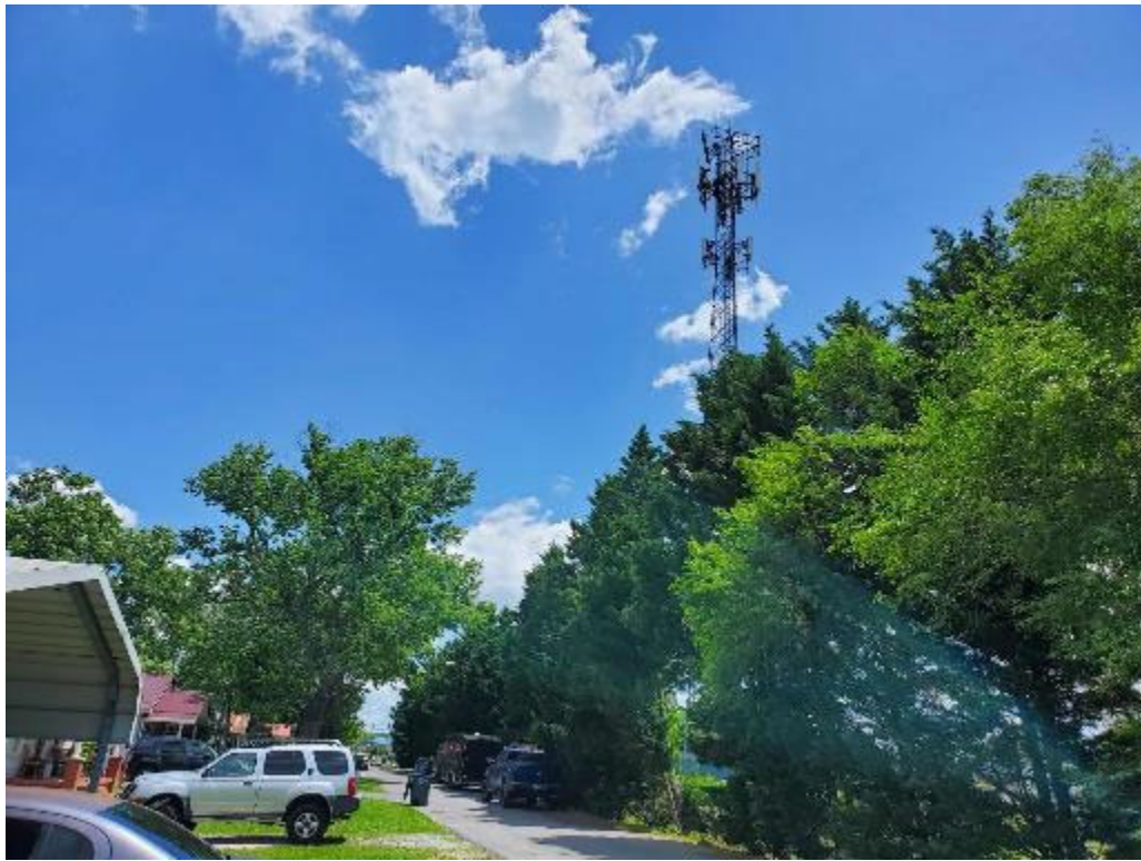
View from 1241 Lomax Street
