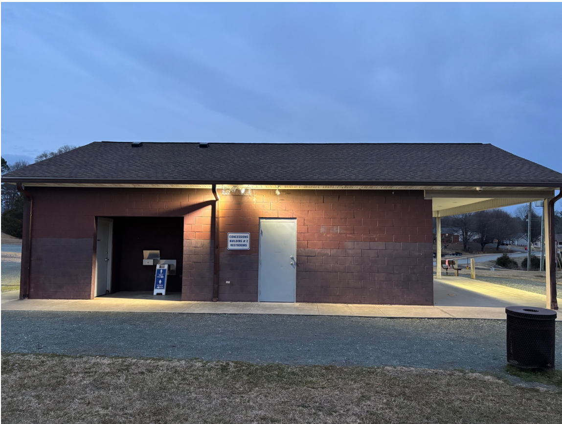
Figure 1 – Current appearance of the concessions building.
