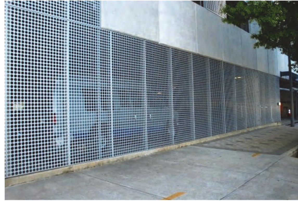
EXTERIOR FINISH 8 (EF-8): PERFORATED SHEET METAL
