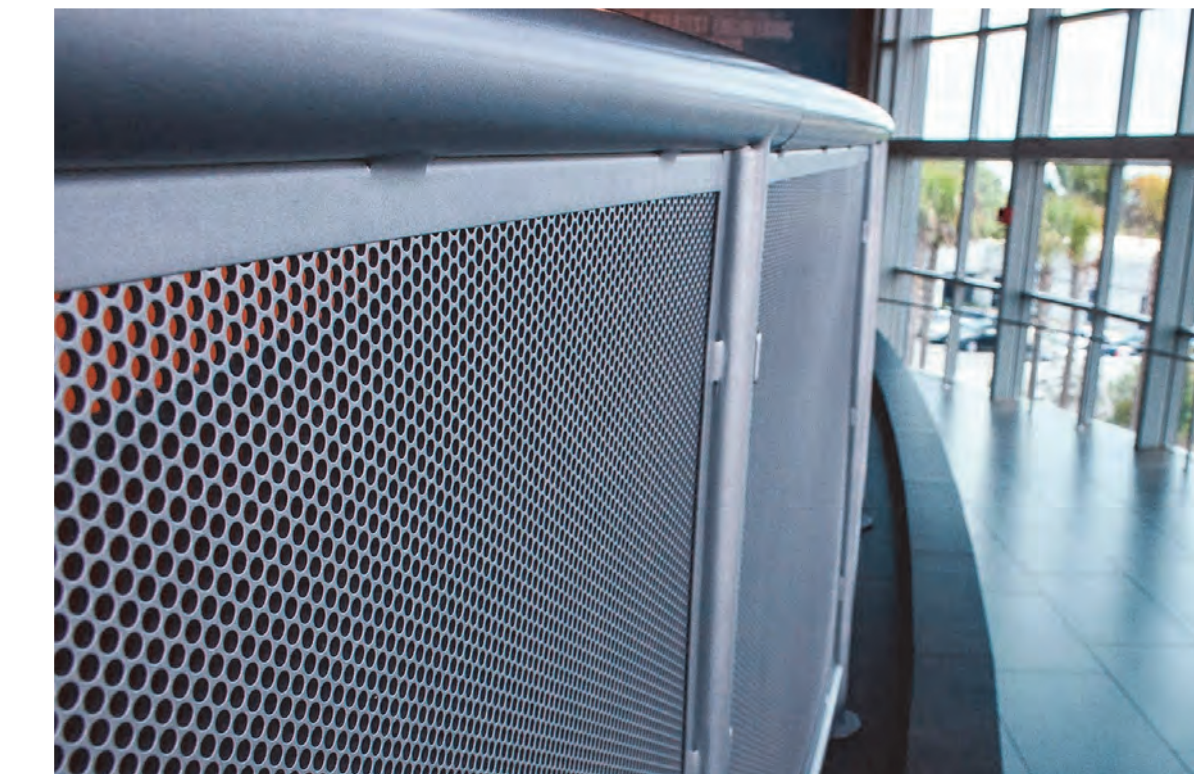
GUARDRAIL 1 (GR-1): MATTE BLACK PERFORATED SHEET METAL
