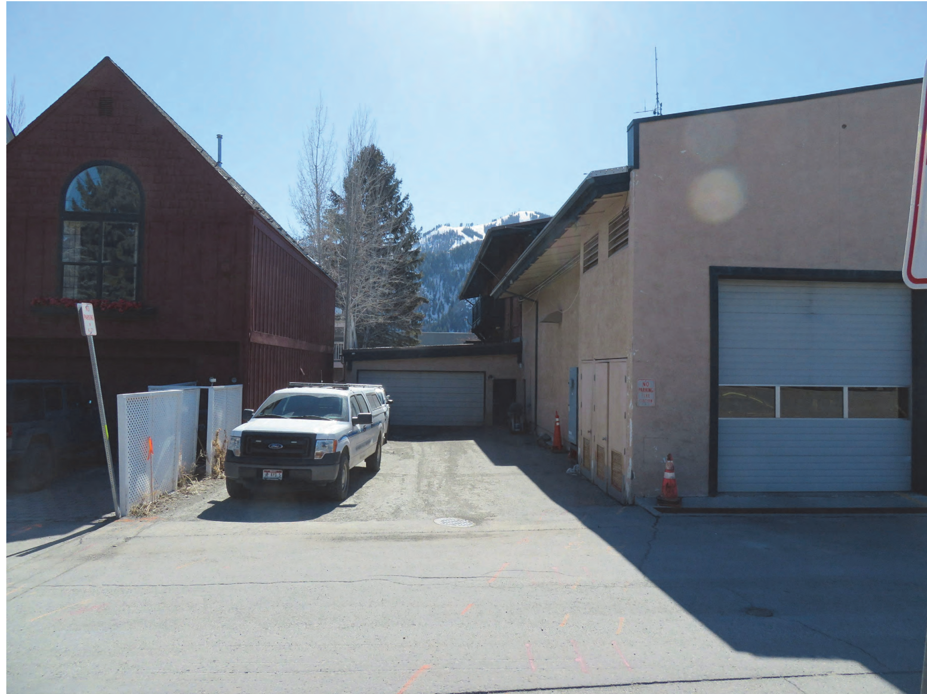
VIEW LOOKING WEST FROM ALLEY ALONG PROPERTY LINE
