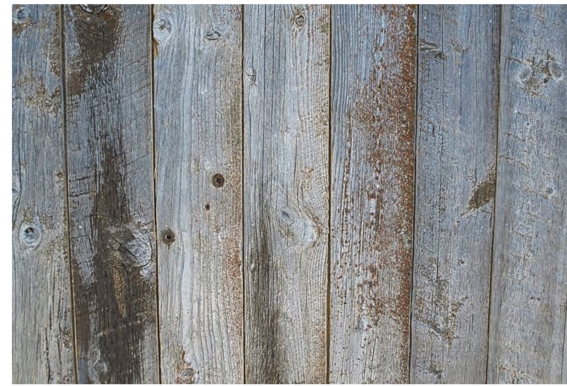
EXTERIOR FINISH 3 (EF-3): WOOD BOARD RAINSCREEN, VERTICAL MONTANA TIMBER PRODUCTS CORRAL BOARD
