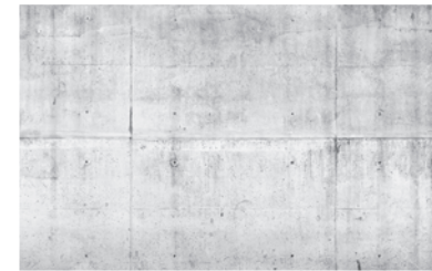
EXTERIOR FINISH 9 (EF-9): EXPOSED CONCRETE
