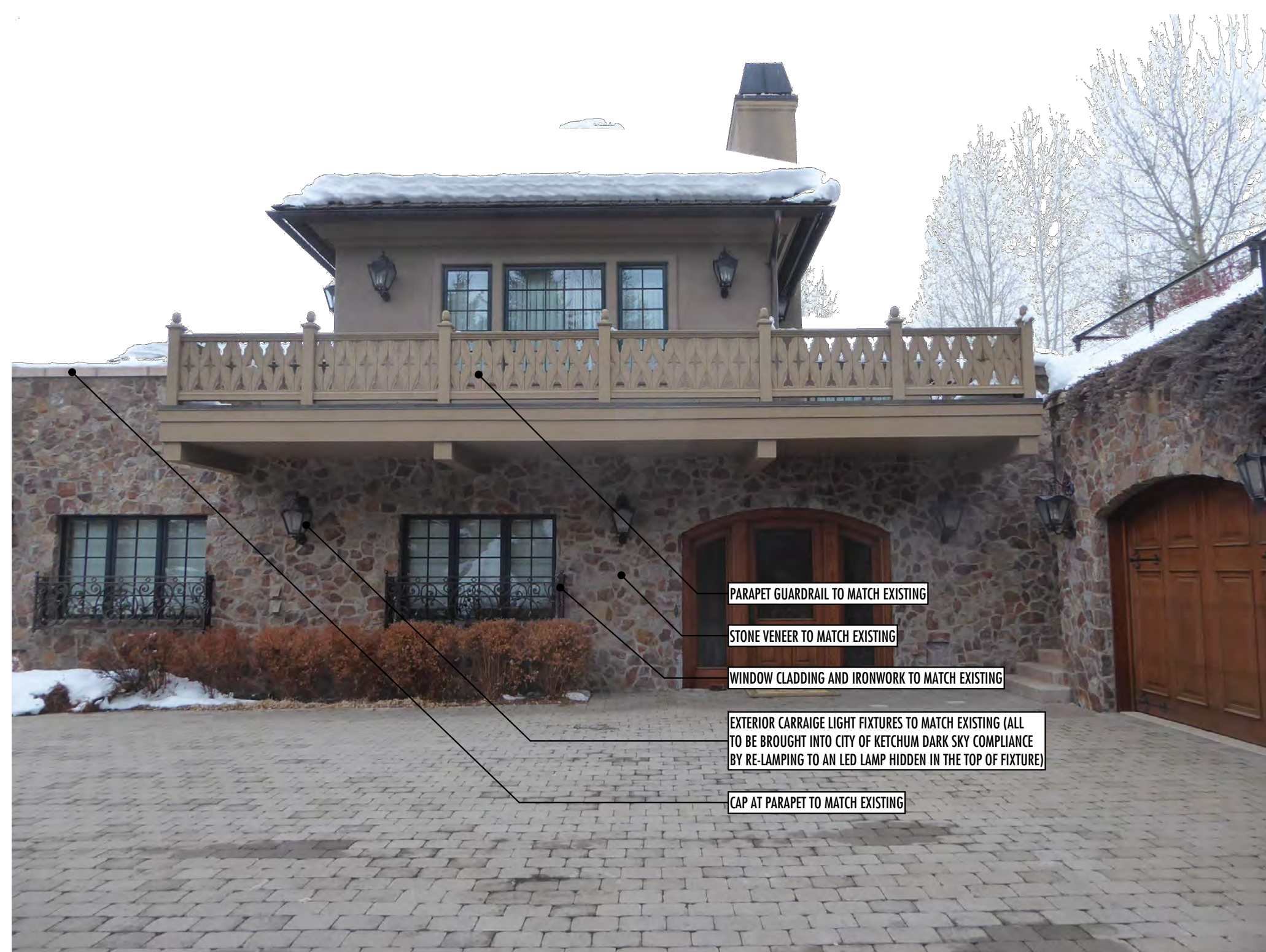
EXTERIOR MATERIALS: TO MATCH EXISTING AS LABELED IN THE EXISTING PHOTO ABOVE
