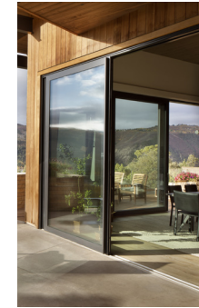
9 MULTI-PANEL SLIDING GLASS DOORS (OPERABLE WALL)
