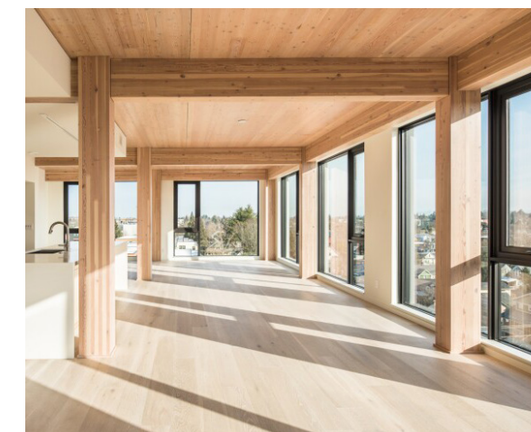
CLT Structure Smartlam, Montana
