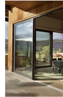
9 MULTI-PANEL SLIDING GLASS DOORS (OPERABLE WALL)
