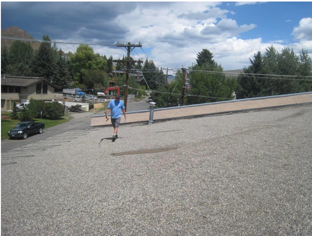
View of two patches at N side of roof; no asbestos detected in 4' x ½" patch (further east); asbestos was detected in 5' x 1' patch (further west).
