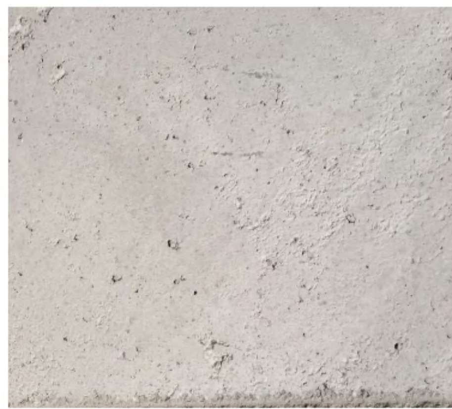
CONCRETE: BASE + STEPS
