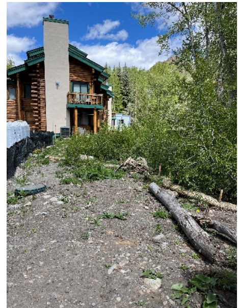
Figure 3: Straw Waddle and Silt Fencing
