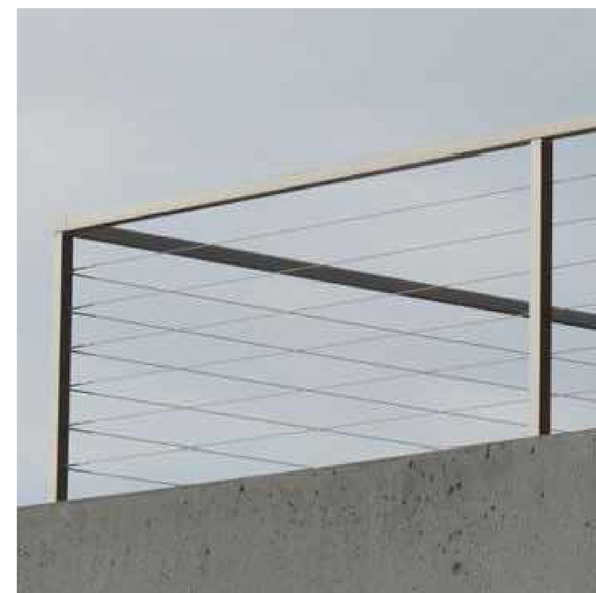
7) Cable Guardrail At exterior terraces
