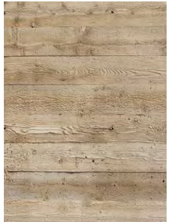
BOARD-FORMED CONCRETE - cast-in-place and stained.
