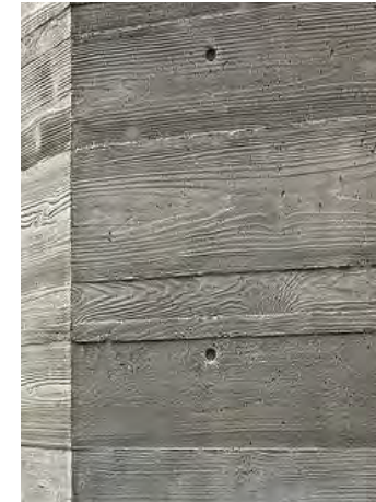
BOARD-FORMED CONCRETE - cast-in-place and stained.
