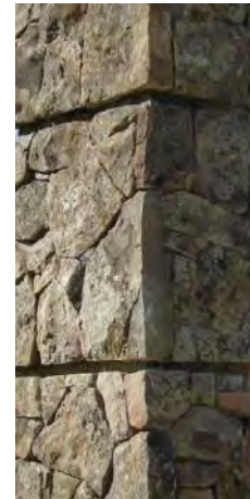
STONE VENEER - Montana Moss Rock natural stone dry-stack lay-up. Stainless steel masonry anchor system.
