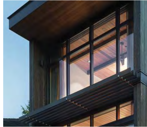
ALUMINUM WINDOWS AND DOORS - powder coated extruded aluminum with Low "E" insulated glass. Basis of Design: Vistaluxe Collection AL Line - Kolbe Windows and Doors. Basis of Design: Reynaers CP155LS Monorail System.
