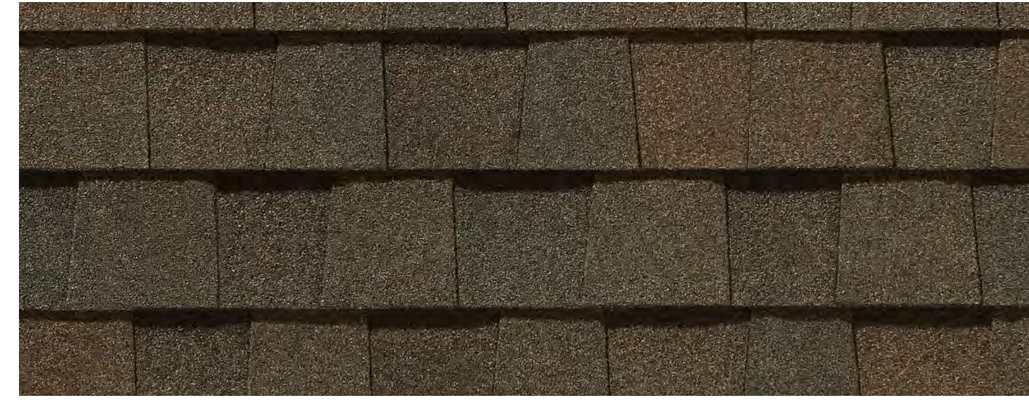
ASPHALT SHINGLE ROOF
