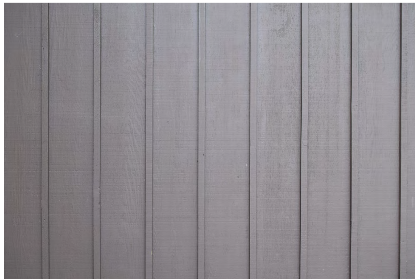
BOARD AND BATT SIDING
