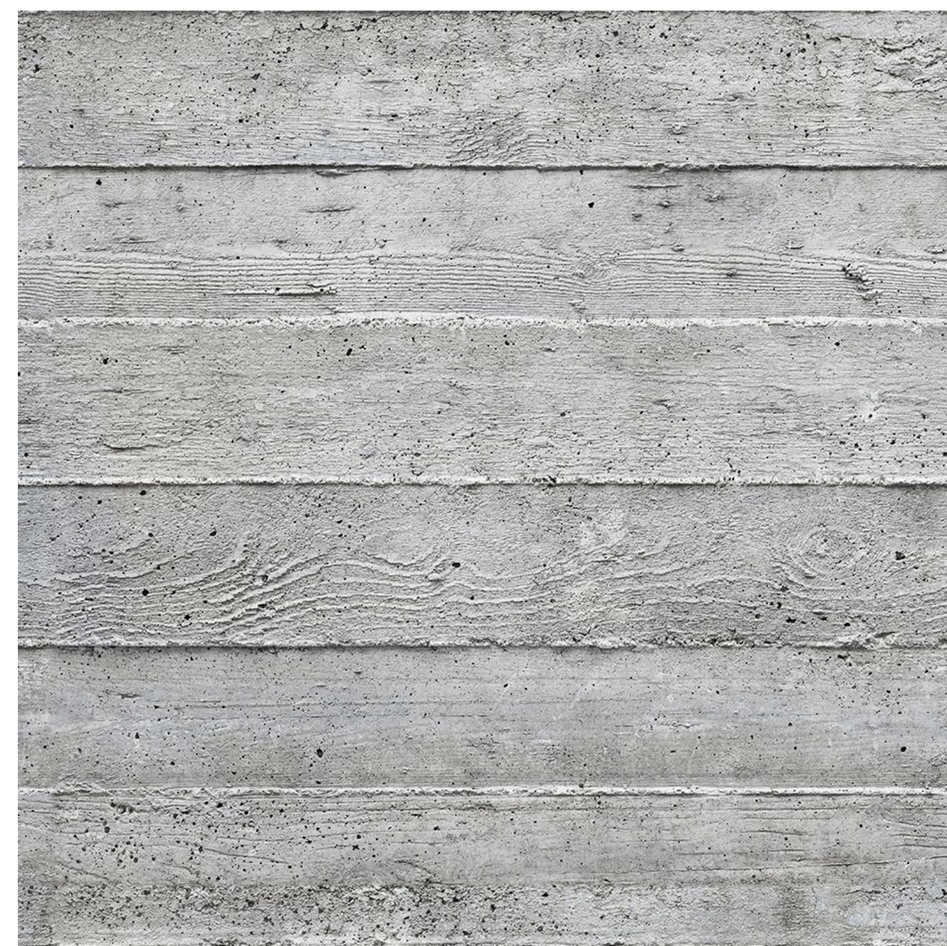
BOARD FORMED FINISH CONCRETE
