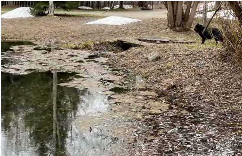
Photo 1 Ditch outfall from pond at 450 Wood River Drive
