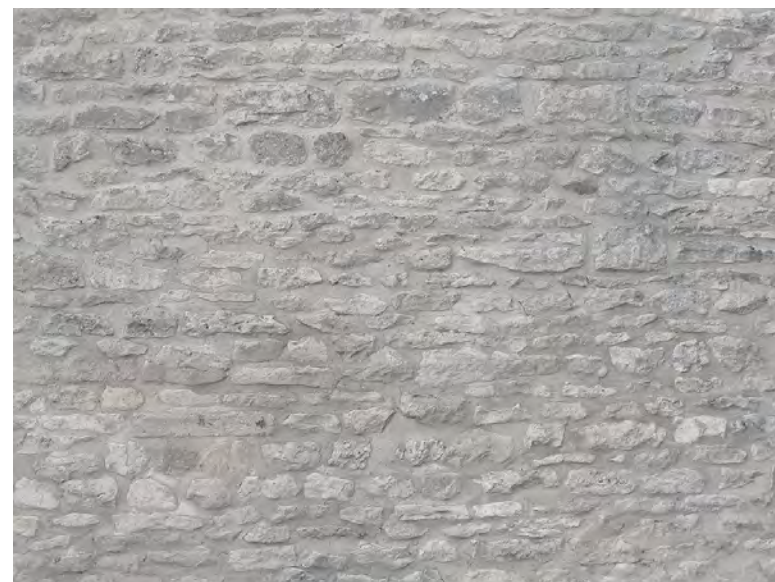
PARGED FIELD STONE: WALLS
