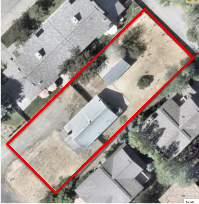
Figure 1: Existing conditions of the subject property
