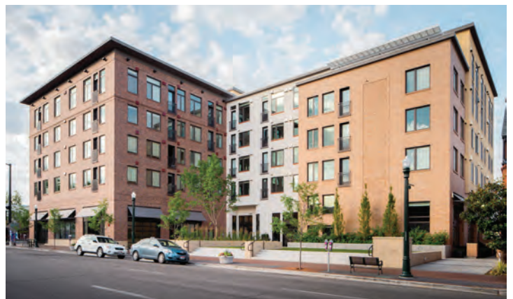
Ash + River Workforce Housing ( upper ) Boise, Idaho
