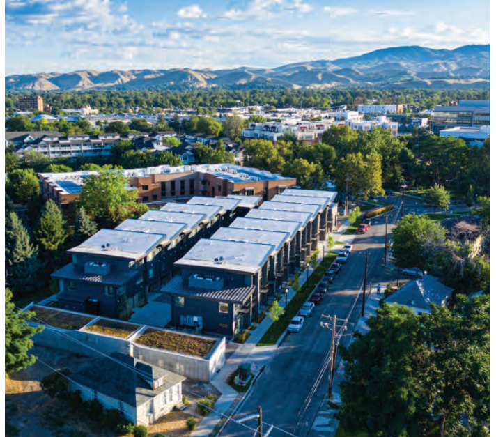
Ash + River Workforce Housing Boise, Idaho
