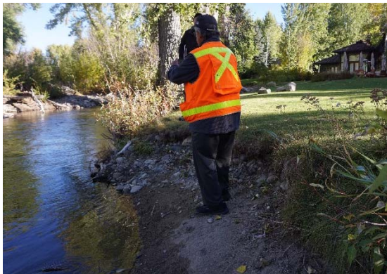
Figure 1: Eroding channel bank in project transition area.
