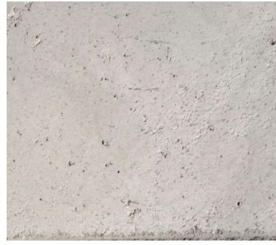
CONCRETE: BASE + STEPS
