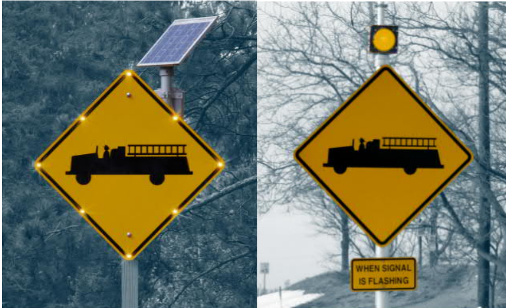
Figure 1. Fire station warning signs with border flashers or beacons. 3
