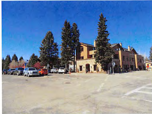
SW CORNER, EAST AVE. & 4TH ST.
