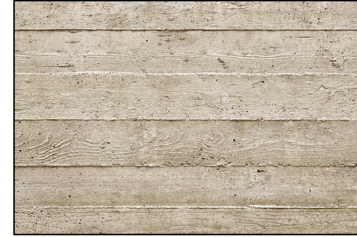
EXTERIOR FINISH 4 (EF-4): TINTED BOARD-FORMED CONCRETE
