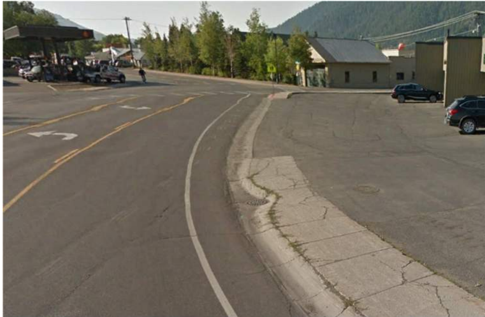
Figure 9. Aged Sidewalk and Large Approach At 10 th & Warm Springs. Source: Google Earth
