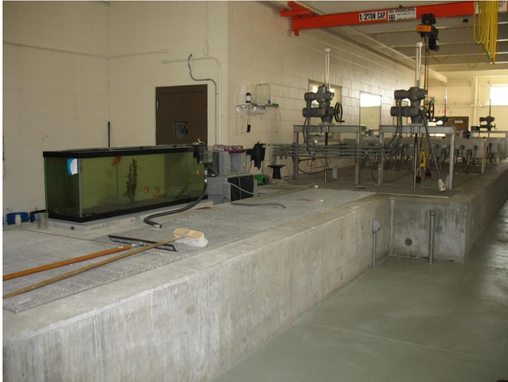
Figure 3-12. UV disinfection system
