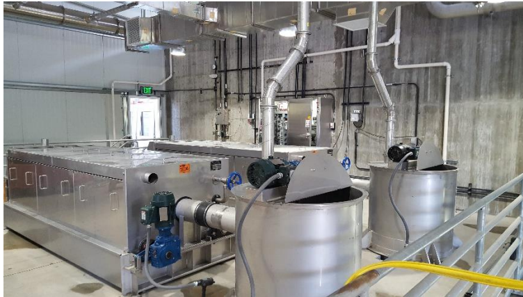
Figure 5-2. Rotary drum thickener
