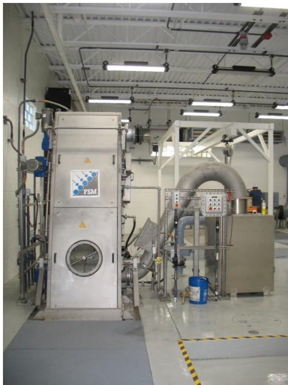
Figure 3-3. Perforated mechanical screen
