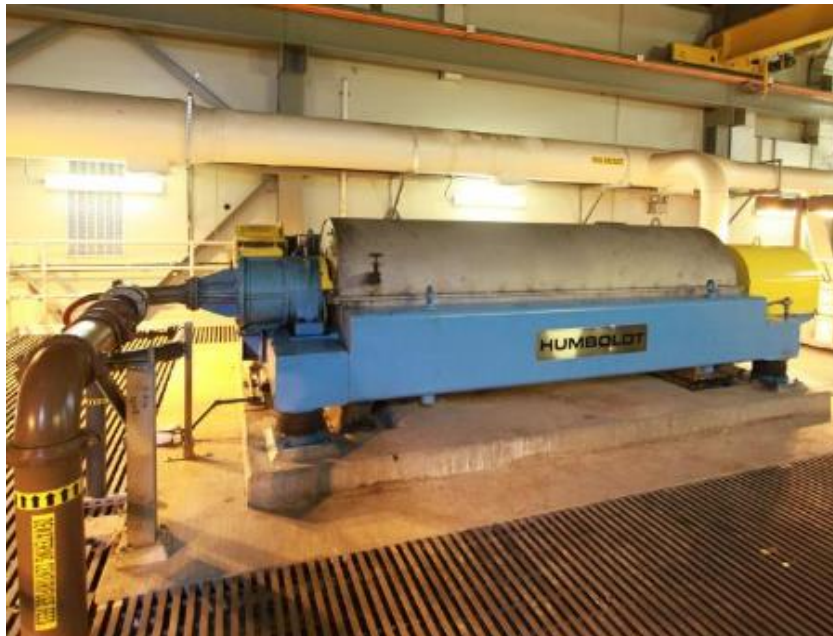
Figure 5-7. Centrifuge at Durham AWWTP in Portland, OR
