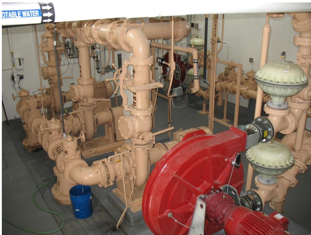
Figure 3-10. RAS and WAS pumping room
