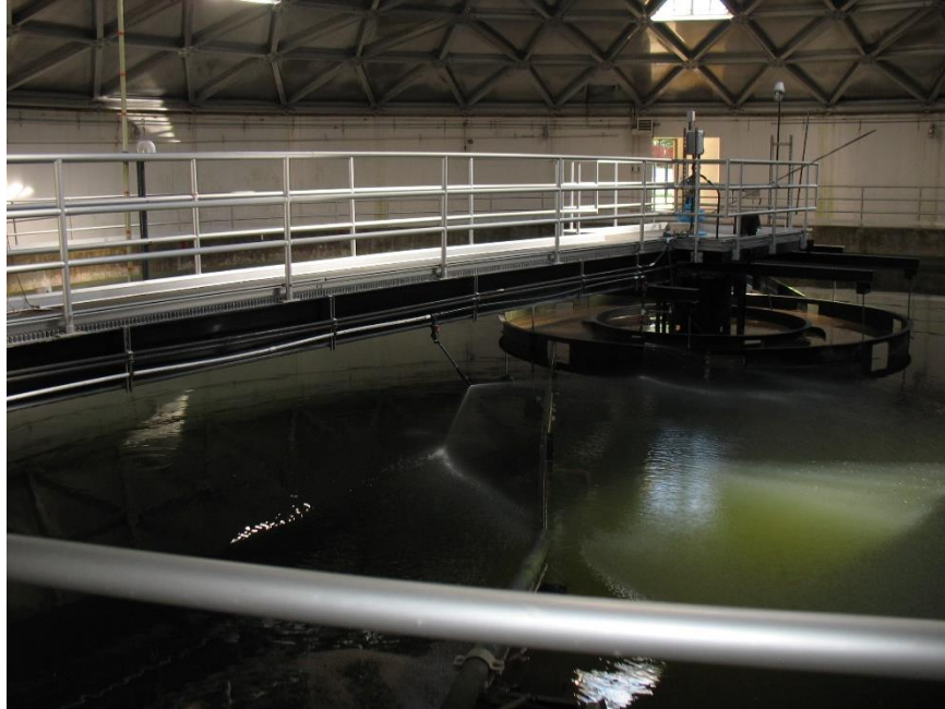
Figure 3-9. Clarifier 1 interior
