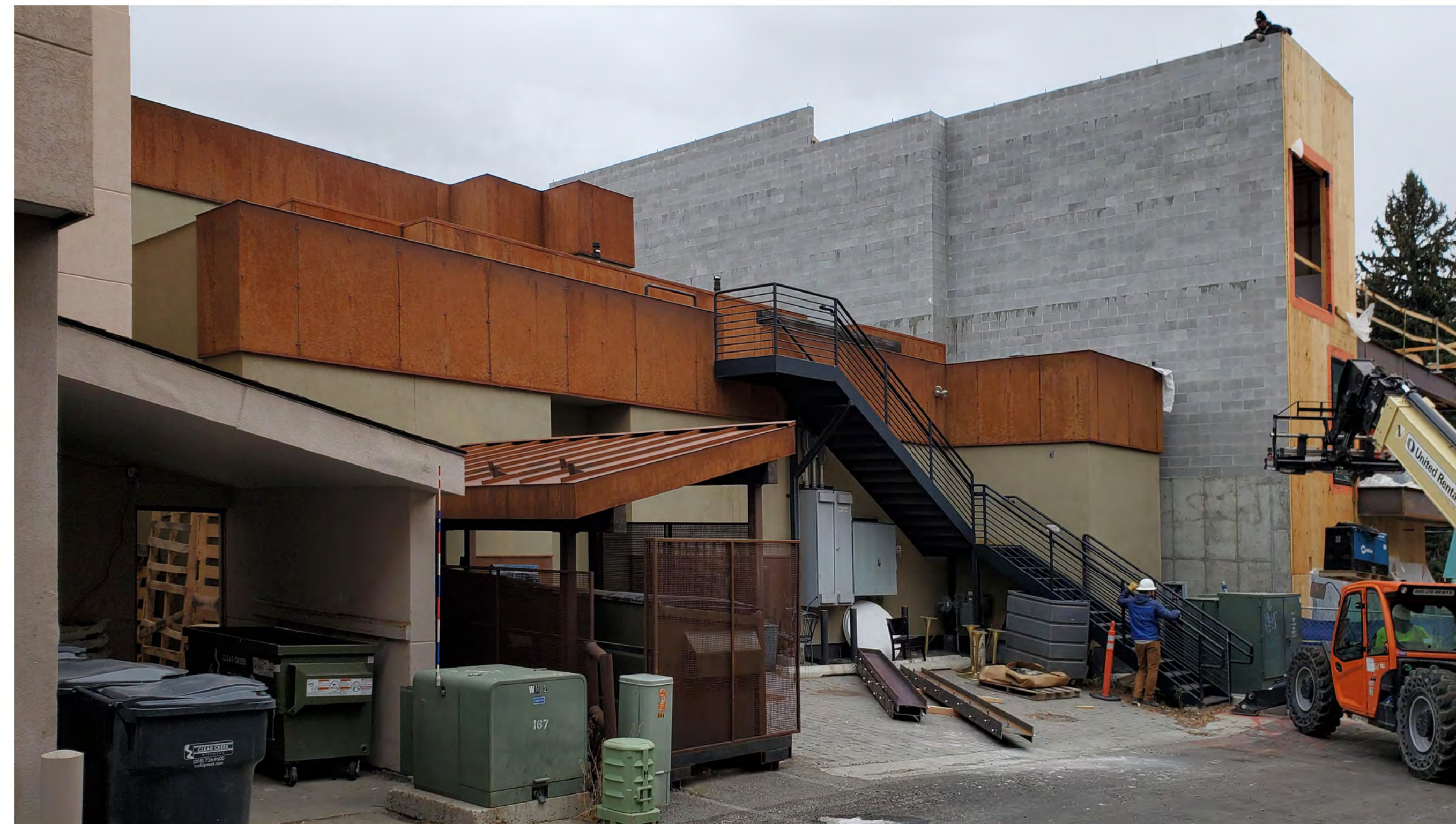
existing north west view
