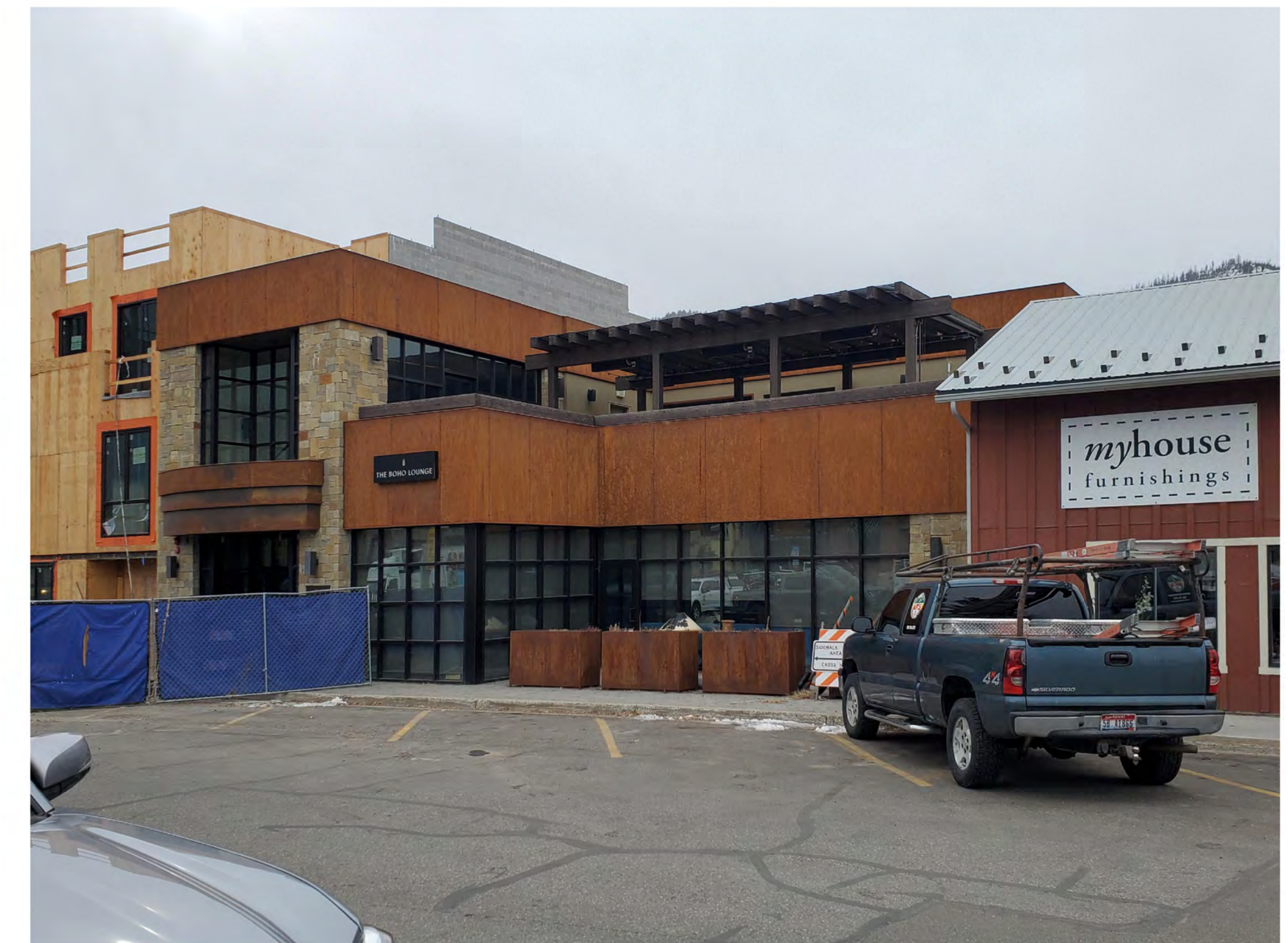
existing north east view
