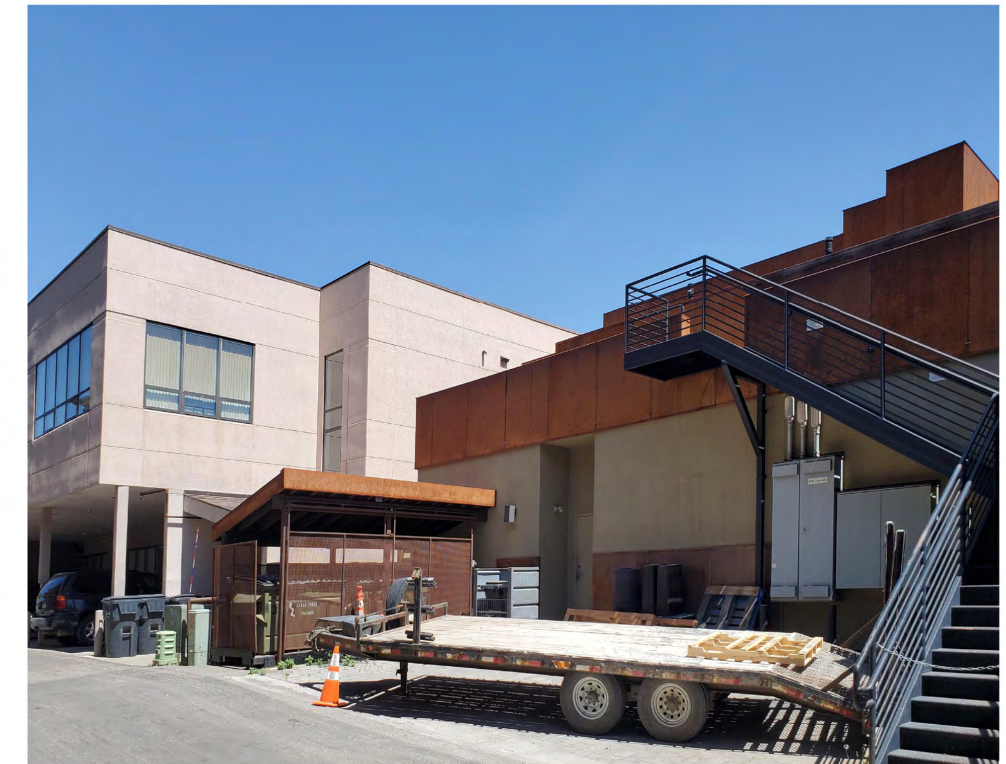
existing south west view
