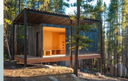
Outward Bound Micro Cabins University of Colorado Denver
