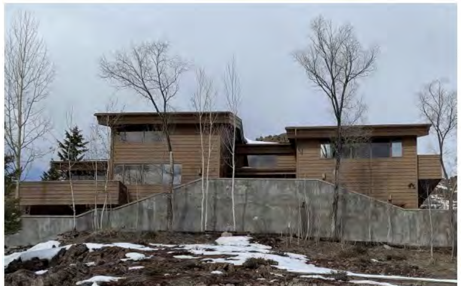
Figure 4: Existing South Side Yard Disturbance (Sheet EX004)
