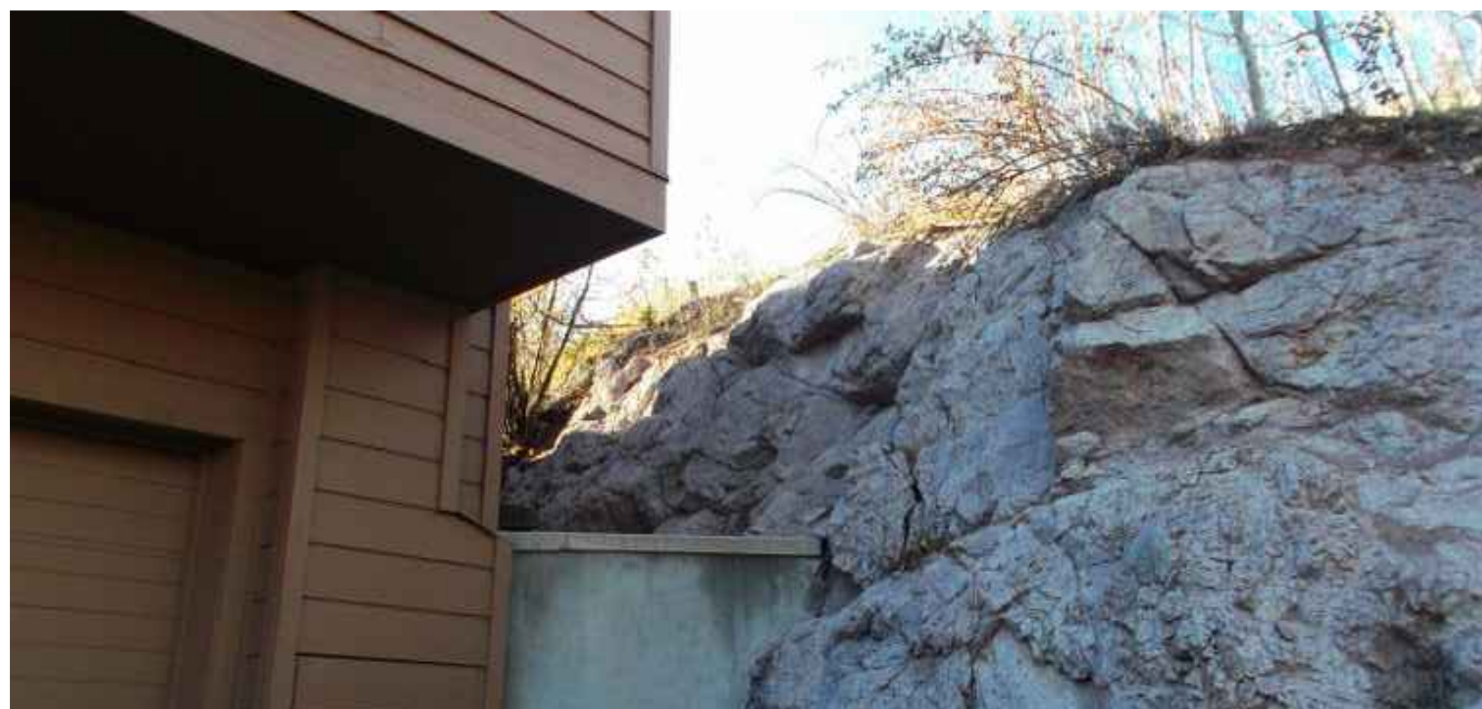
2) View from driveway
