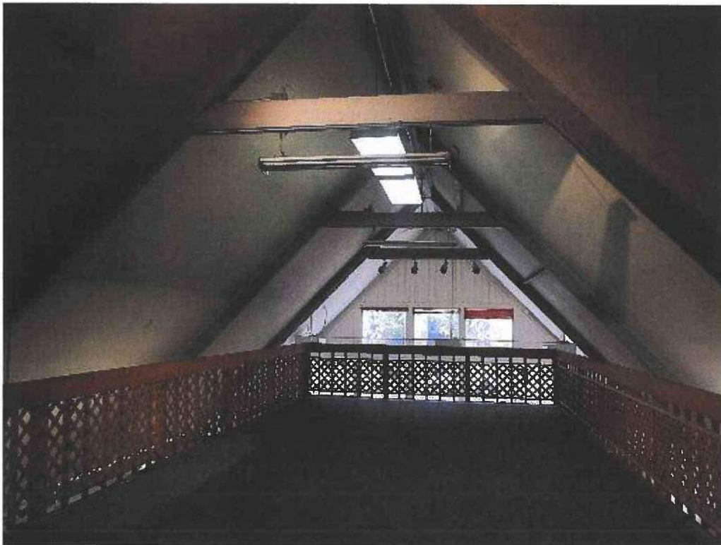
Photo 22: View of mezzanine
