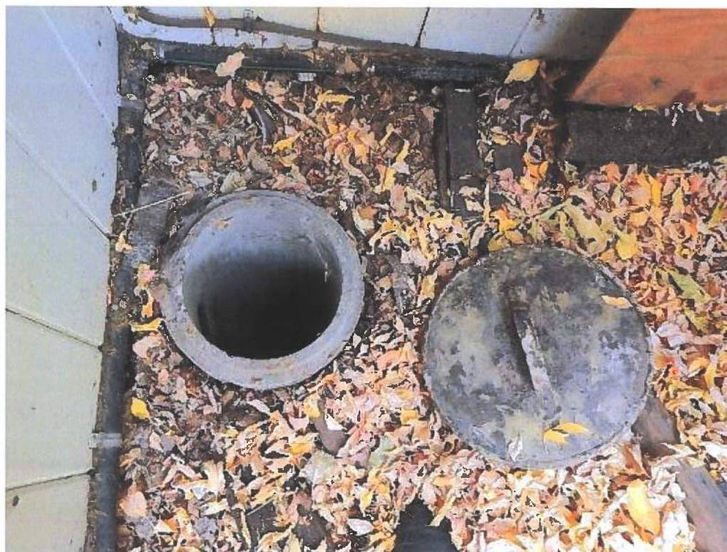
Photo 10: View inside concrete conduit behind building Note: metal valve key likely for water shut off
