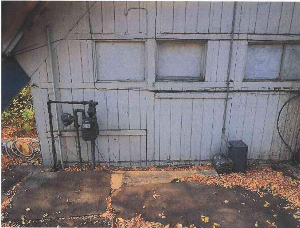
Photo 11: Outside rear of subject building
