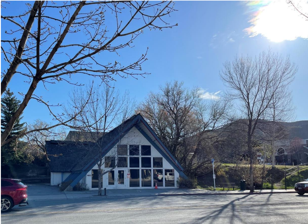
1. Front of Building
