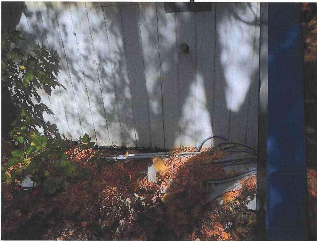
Photo 12: Outside east corner of building
